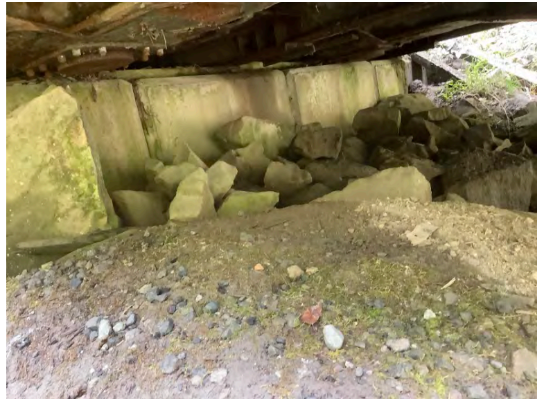
Left Bank Abutment when facing downstream
