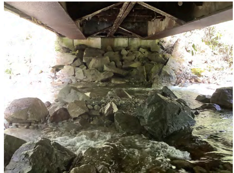
Right Bank Abutment when facing downstream
